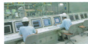
N-1号抄紙機制御室 Control Room of Paper-Making Machine N-1
